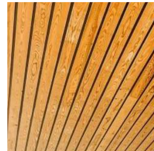
WOOD CEILING & WALLS within covered plaza connection
